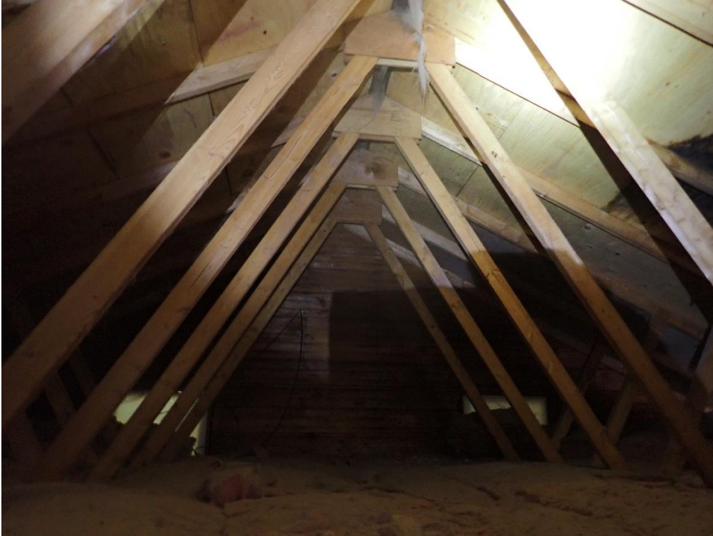
Photo 43: Addition – Roof Framing Typical Condition
