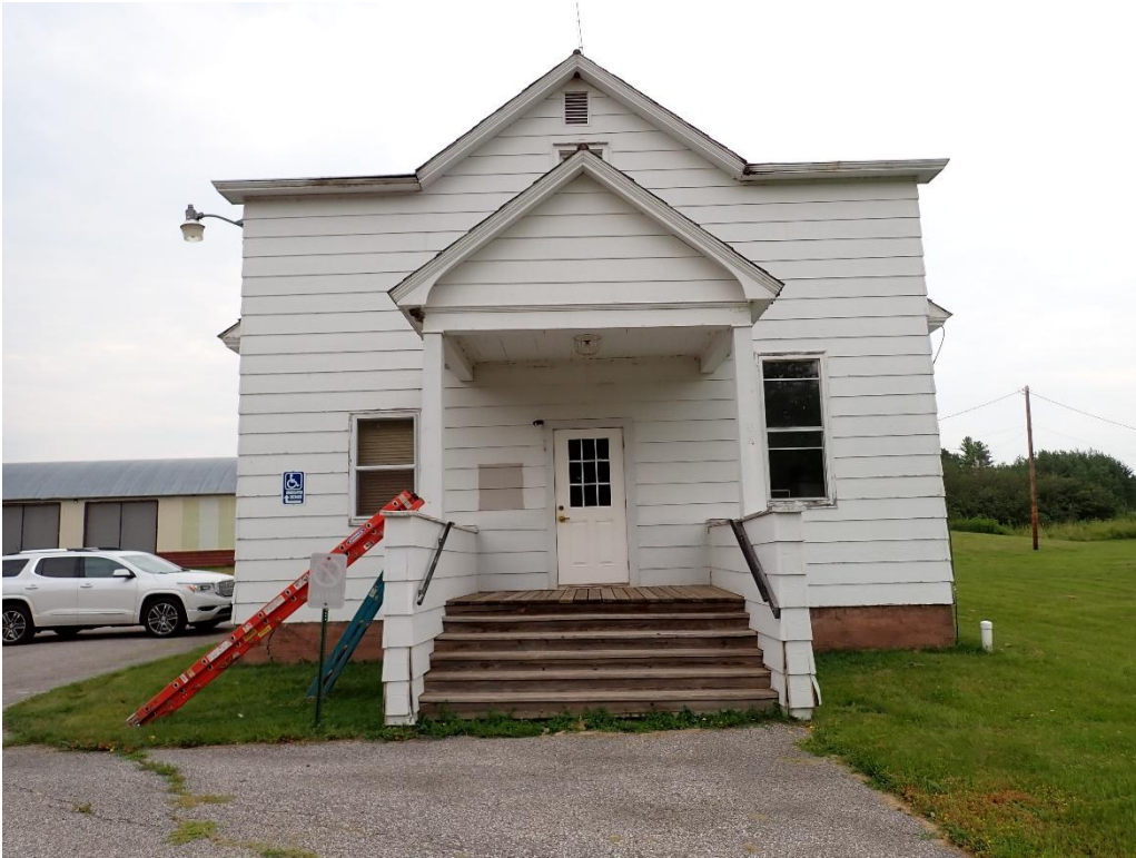
Photo 25: Building Elevation Looking North – Front Entrance Porch
