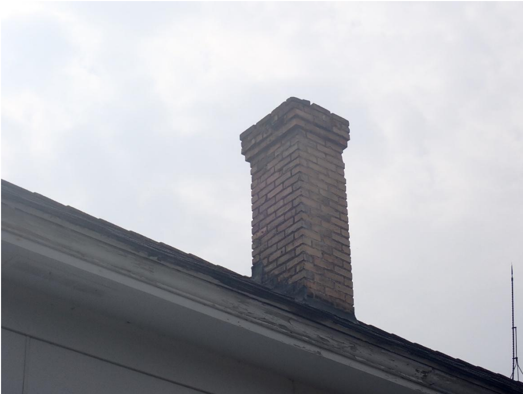
Photo 45: Chimney – Looking SE
