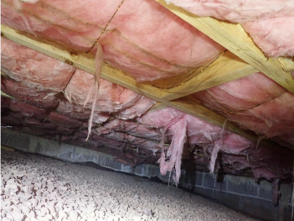
Photo 41: Addition – Typical Floor Framing
