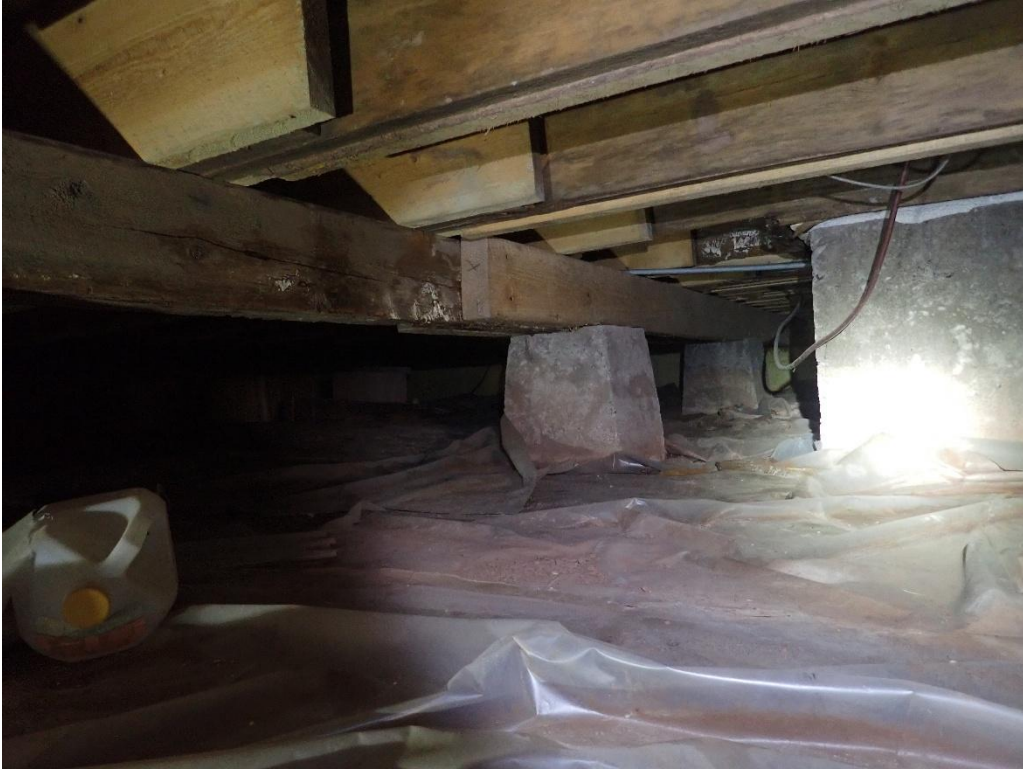
Photo 19: Sistered Beam (P6-P7)
