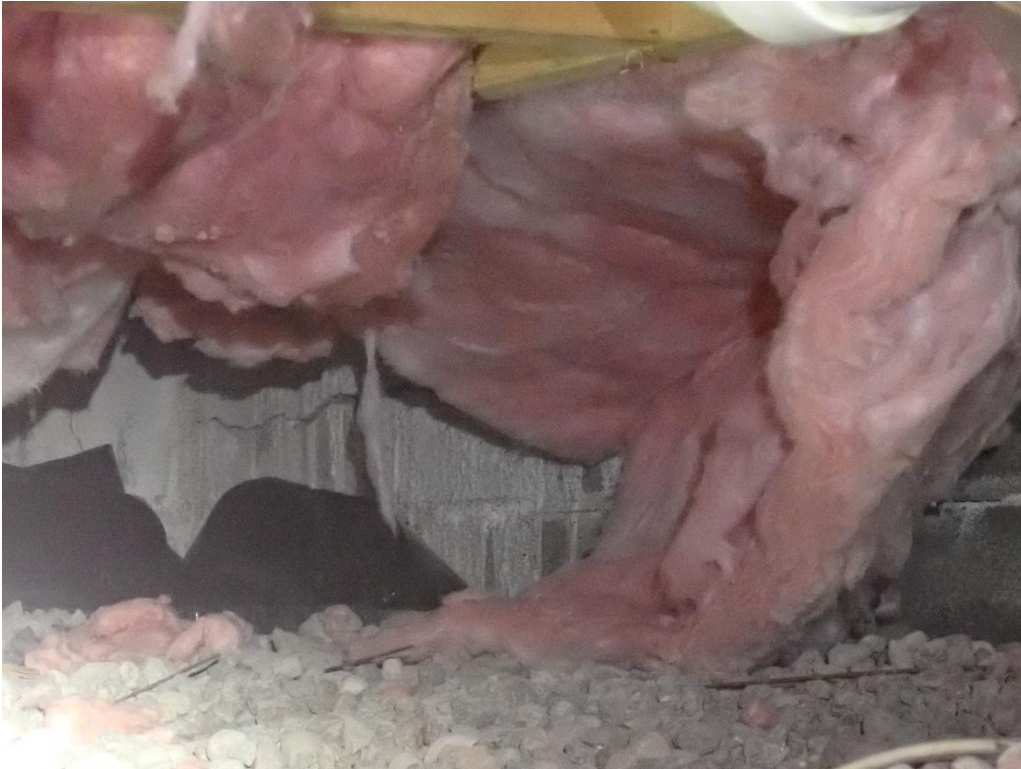
Photo 37: Addition – Horizontal Cracking through the CMU at the West Wall
