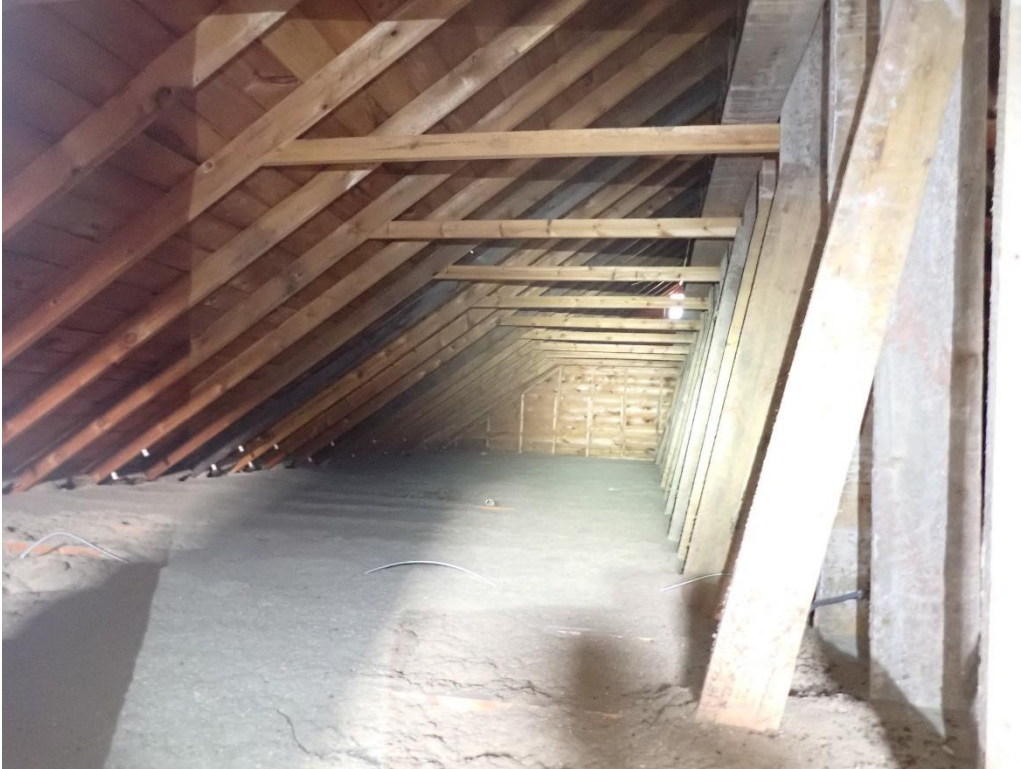
Photo 23: Roof Framing – Original Building
