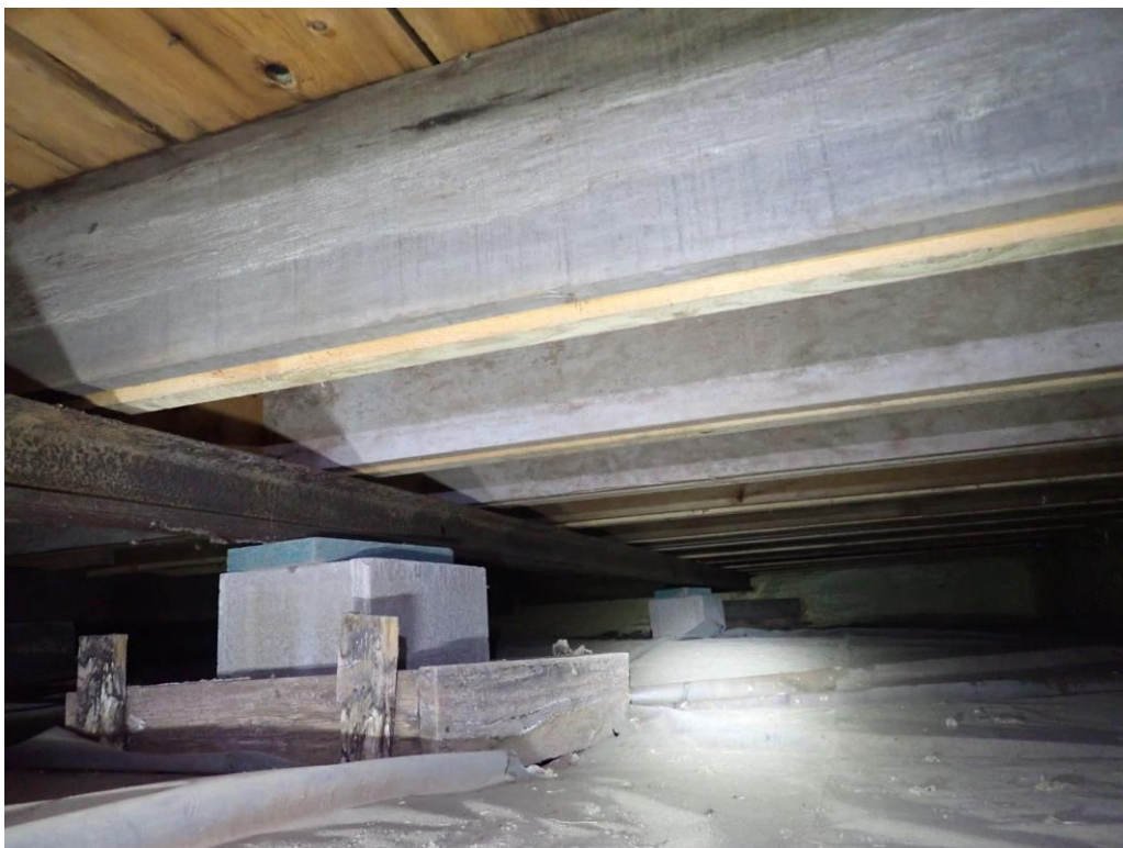
Photo 18: Typical Floor Framing Condition (East)
