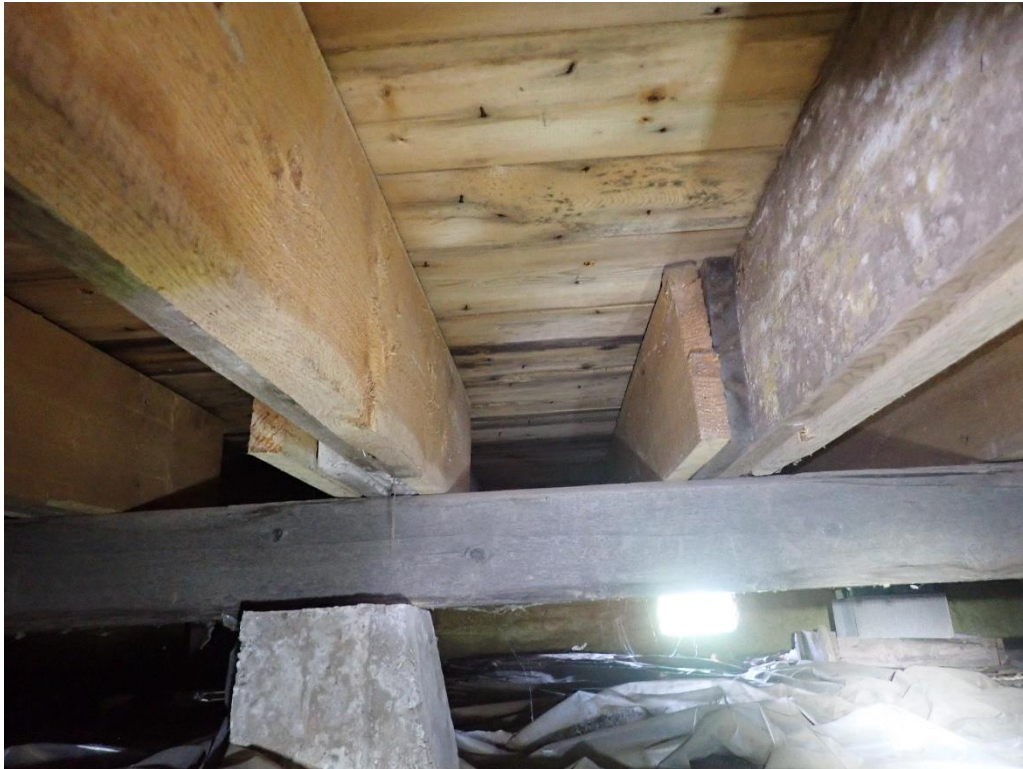
Photo 17: Typical Floor Framing Condition – Checks in Timber Beam (West)
