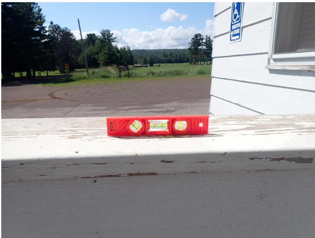
Photo 28: Porch Sloping Towards North
