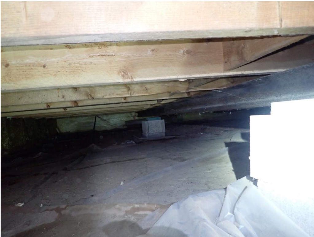
Photo 16: Typical Floor Framing Condition (West)
