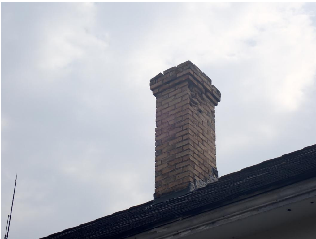
Photo 46: Chimney – Looking NE
