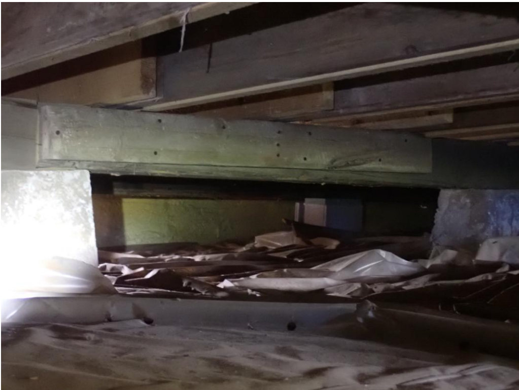
Photo 20: Sistered Beam (P4-P5)
