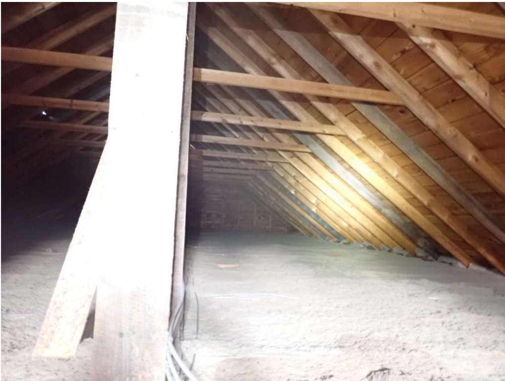
Photo 22: Roof Framing – Original Building
