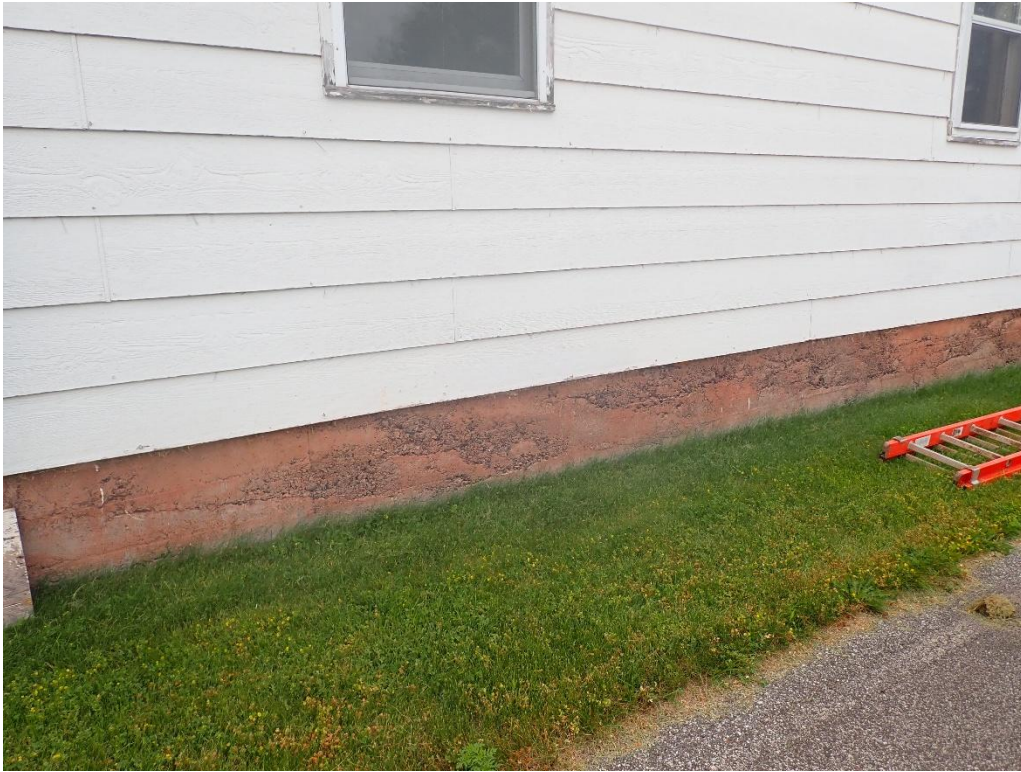
Photo 7: West Foundation Wall
